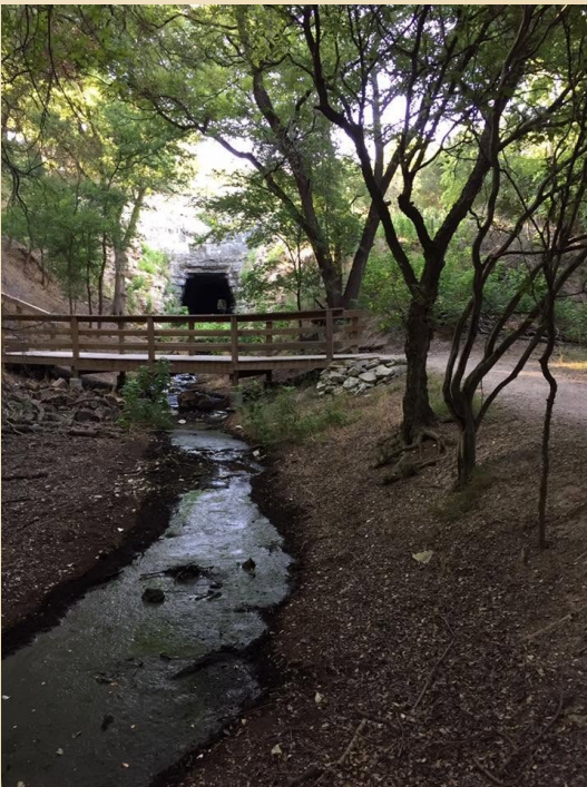
Old Tunnel SP
