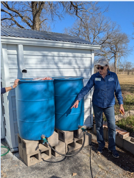
Kim points out how two barrels connect at the bottom so they fill equally
