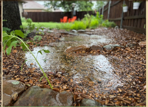
Creek bed berms slowing water runoff
