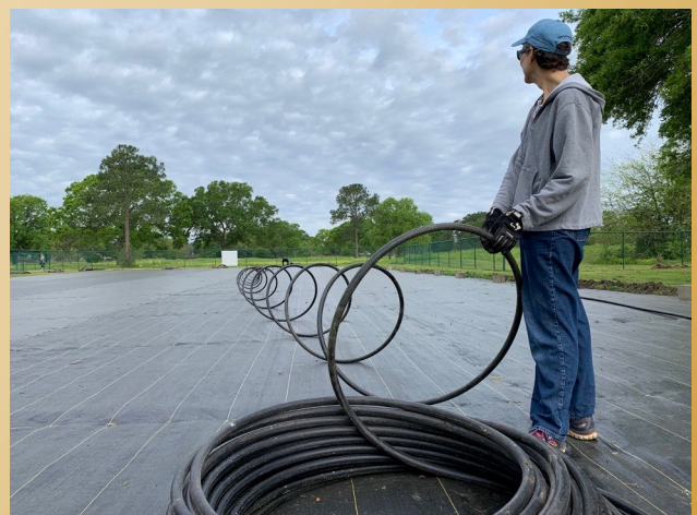
Installing an irrigation line
