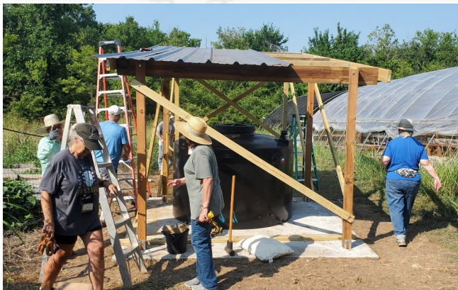
2020 class project—installing the roof
